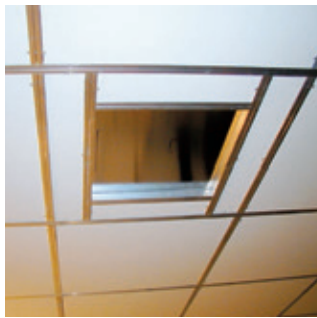
Shielded hatch for ceiling
